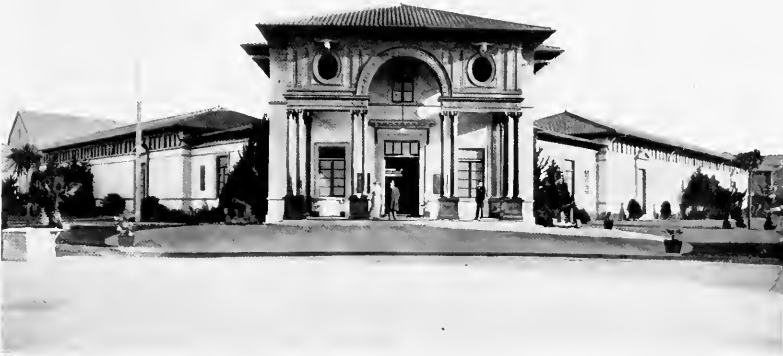
THE PHILIPPINES BUILDING
